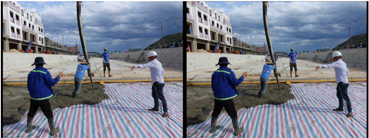
Robert McRostie - Laying Concrete.jpg
